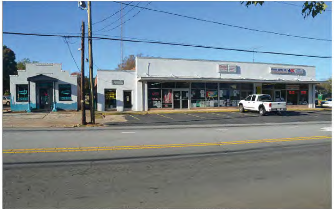
Figure 48: Brown Supply (existing conditions)
