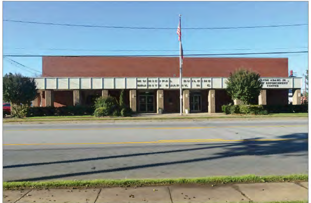
Figure 42: Municipal Center (existing conditions)
