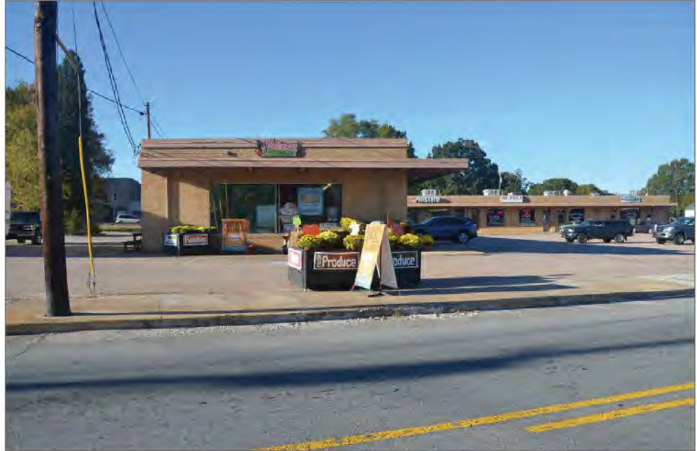
Figure 38: Brinkley Center (existing conditions)
