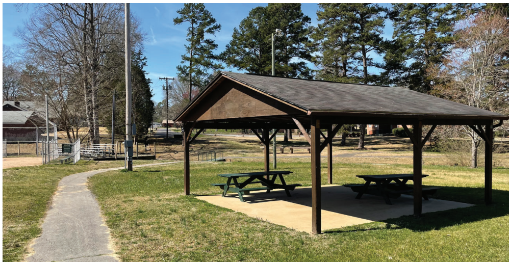
Shelter lacks paved accessible route
